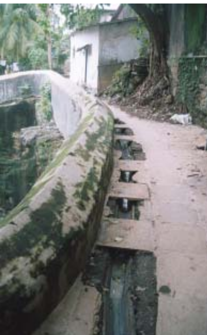
DRAIN AROUND THE CAVE
