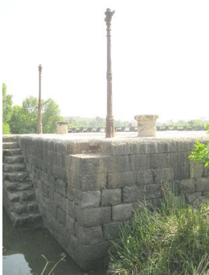
002 Pier in the black basalt stone masonry
