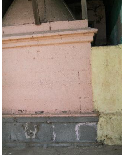
008 Black basalt stone plinth of the Mandir
