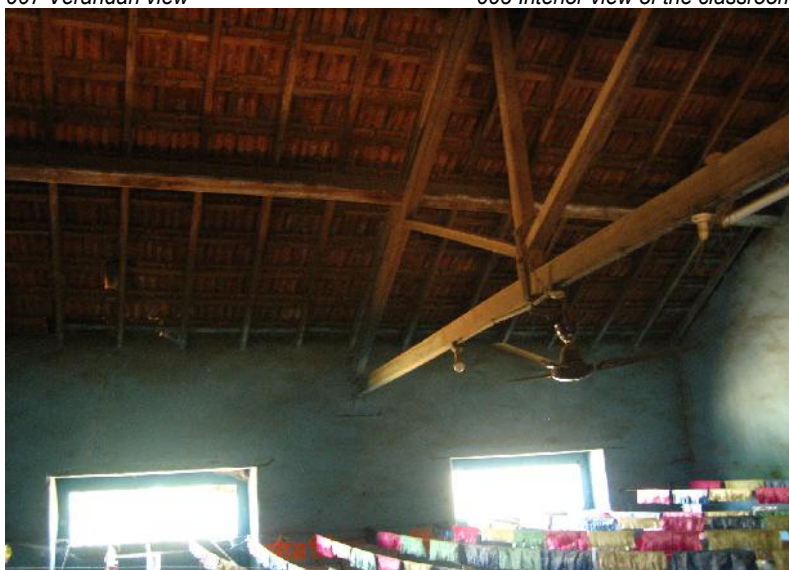
009 Interior view of the classroom showing the roof trusses
