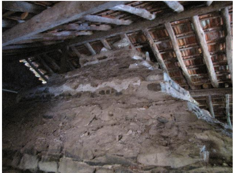
006 View of the pyramidal shikhar with manglore tiled wooden roof above
