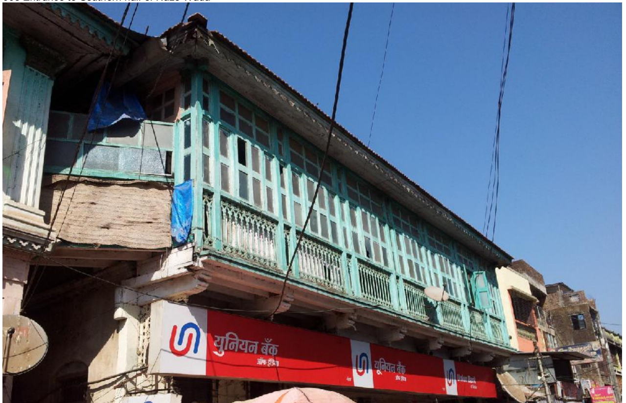
006 Northern half of Naze Wada -Gallery at the first floor enclosed with the decorative cast iron railing, set of wooden posts and wooden windows
