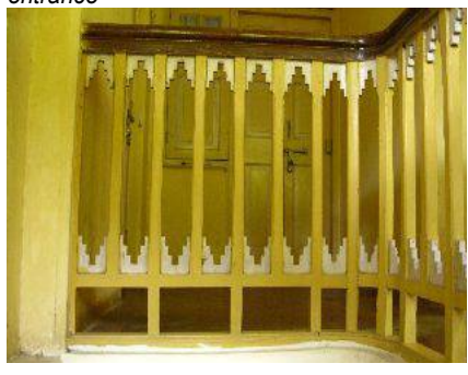
010 Wooden staircase well railing
