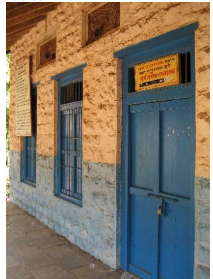
014 Typical teakwood door with double shutter and ventilator above
