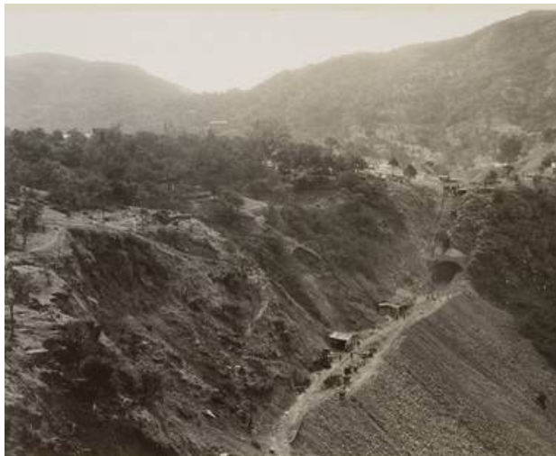
008 Bhor ghat re-alignment under construction. View from top of tunnel 2 towards tunnel 1
