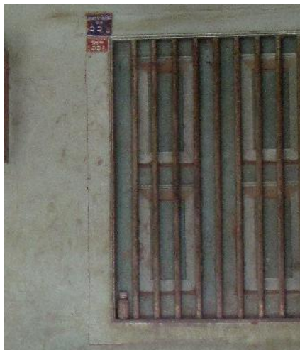
010 Iron rods embedded in the window frame
