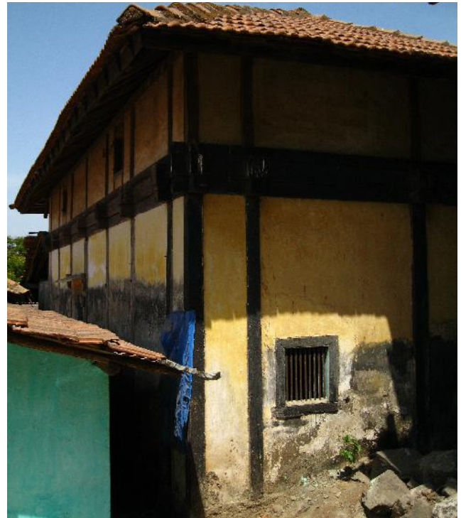
005 North West exterior view of the wooden post and beam framework and lime plastered walls
