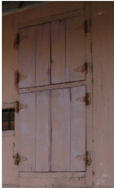
011 Typical teakwood window split in two horizontal halves with double shutters
