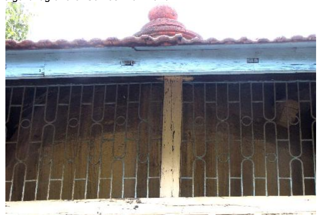
021 Manglore tiled roof covering dome of the garbhagruha
