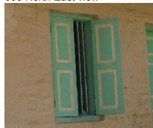
005 Typical wooden window with double shutter
