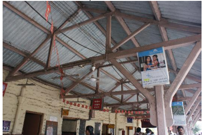
011 Wooden trusses, posts and brackets on Western platform
