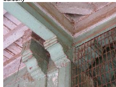
017 Decorative wooden brackets supporting the beam
