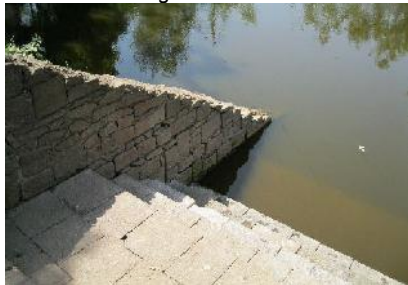
005 Stone wall lining of the ghat and steps
