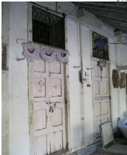
014 Typical wooden door with double shutter and ventilator above
