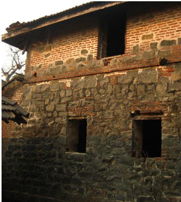
006 South side stone & brick composite masonry wall
