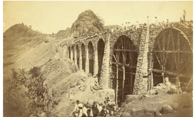
005 Construction photo of a viaduct on the Bhore ghat
