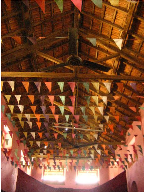
010 Roof Trusses in the classroom
