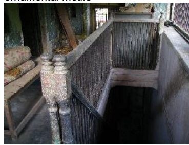
012 Internal staircase with the wooden railing and ornate newel post
