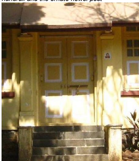
012 Typical wooden entrance door with double shutter
