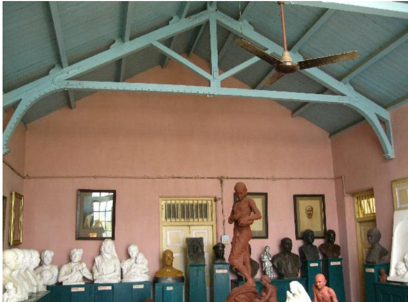
015 Sculpture display in the first floor studio covered by the sloping roof supported with typical wooden king post trusses
