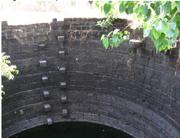
002 Internal stone steps along the well's inner wall surface
