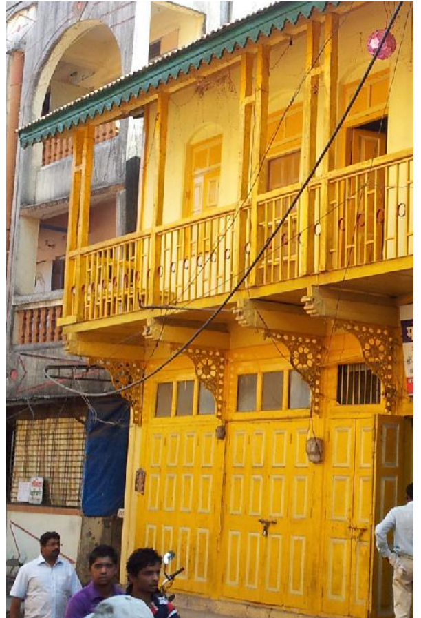
003 Facade showcasing the wooden folding shutters, cast iron brackets and timber beams supporting the extended gallery and the cast iron railing fixed in set of wooden posts.
