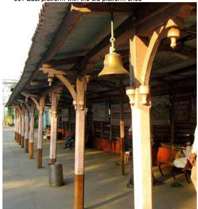
003 Wooden posts and ornamental brackets on Eastern platform
