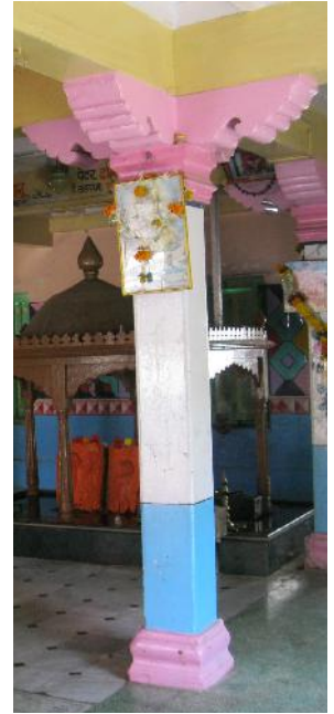
013 Wooden post with the stone base
