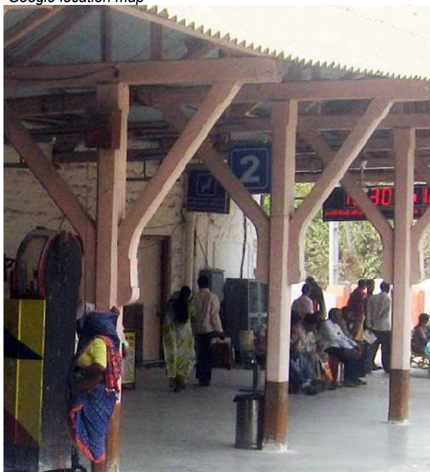
002 Wooden posts and brackets on Western platform
