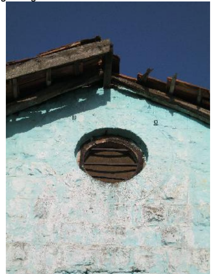
006 Circular ventilator in the gable wall
