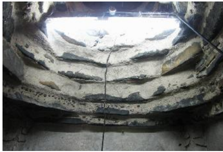
004 Shikhara interior view of the stone corbelling
