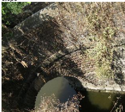
006 Arch at the junction of the well and the tank
