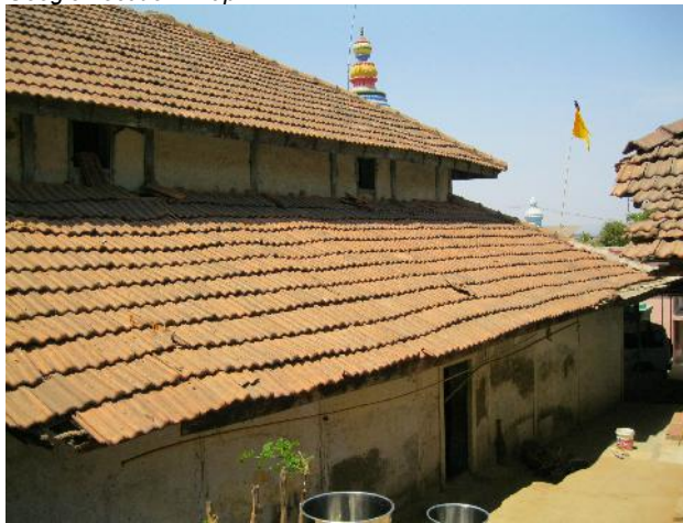
002 Exterior view of the hipped and lean to roofs
