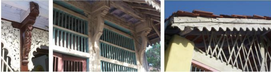
Figure 12 Wooden Brackets in Ganpati Mandir (left), Brackets and Jalis in Temple Street (centre) & Typical Roofing style (right)
