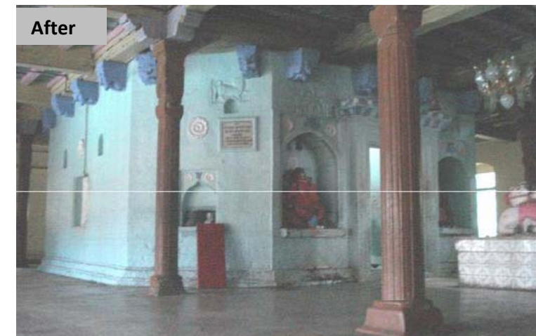
Stone Walls of the Garbha Griha have been painted with layers of oil paint over the period of years. Periodically wall surfaces of the temples are painted as regular maintenance.
