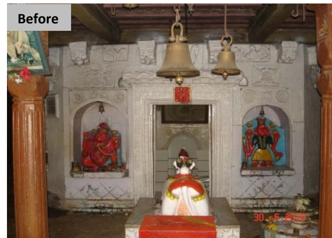
Stone Walls of the Garbha Griha have been painted with layers of oil paint over the period of years. Periodically wall surfaces of the temples are painted as regular maintenance.
