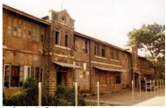
Grade III: Railway Housing
