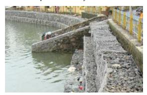
Newly made steps of stone masonry leading to water
