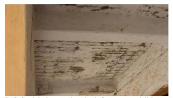
R.C.C. slab damaged and reinforcement visible
