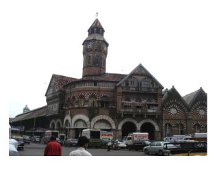
The building adopted an interesting construction of cast iron columns and large roof trusses to achieve a large span interior space. The outer shell was in stone masonry, employing Malad and Kurla basalt and Porbunder limestone. The red stone used rather sparingly in the arch voussoirs, was quarried in Bassein, while the gable end was in a half timber construction, reminiscent of Elizabethan buildings in England.
