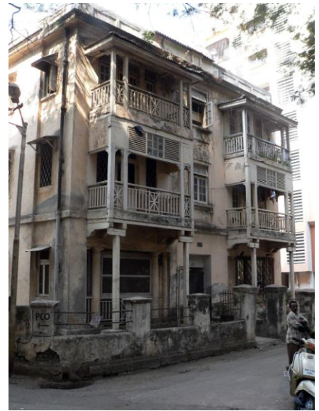
View of front facade
