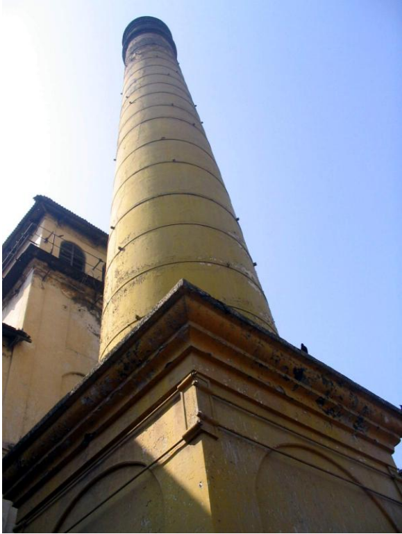
View from bottom of the Chimney
