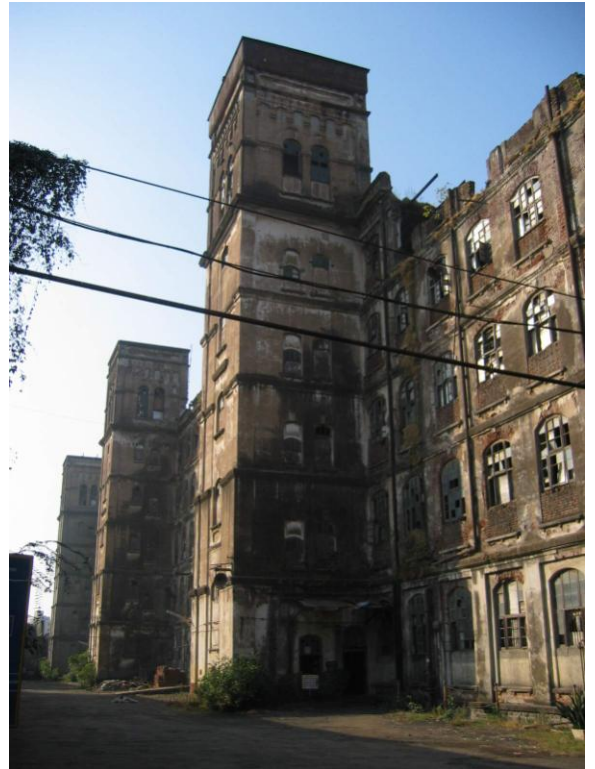
View of the Spinning Structure
