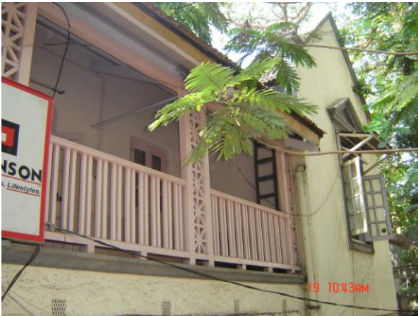
View of balcony having wooden railings
