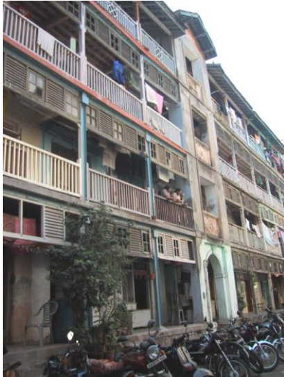
Internal view Krishna Chawl Precinct
