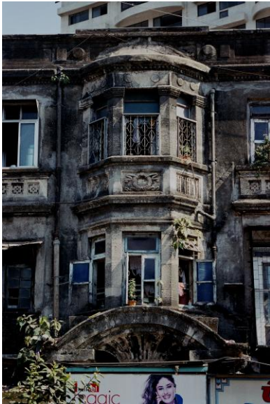
Decorative balconies with pilasters
