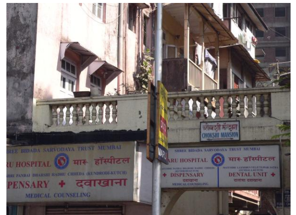
Entrance Bridge detail
