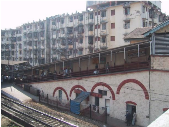
View of the station platform from the bridge.
