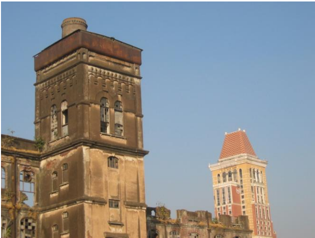
View of staircase shaft
