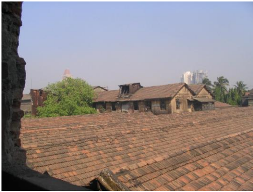
Roofscape, Jam Mills
