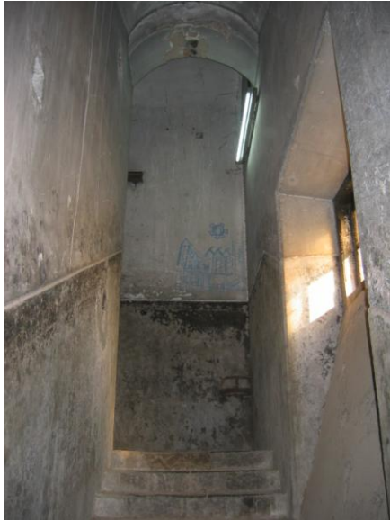
View of staircase
