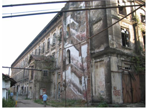
Structures follow a careful blend of Vernacular and Industrial architectural character
