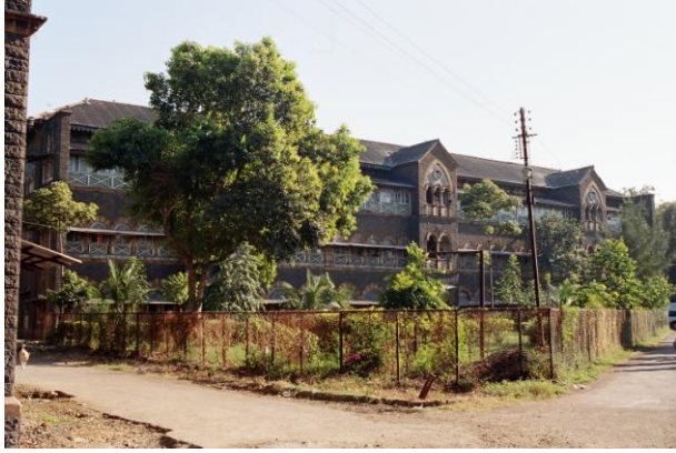
View of Railway Board Building from internal road
