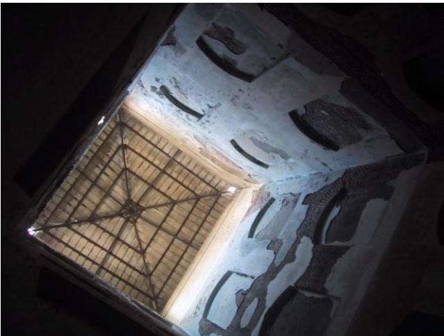
Internal view of Dust Chimney
