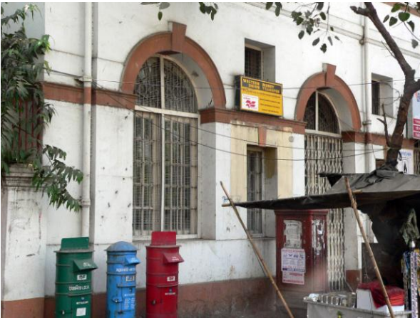
Semi-circular arches with simple keystone
