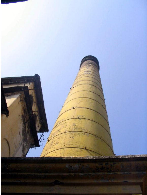
Goldmohur Mills - Chimney
