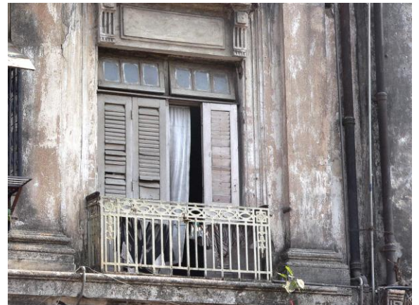
Louvered wooden doors
