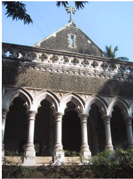
Decorative entrance canopy, with decorative equilateral arches
