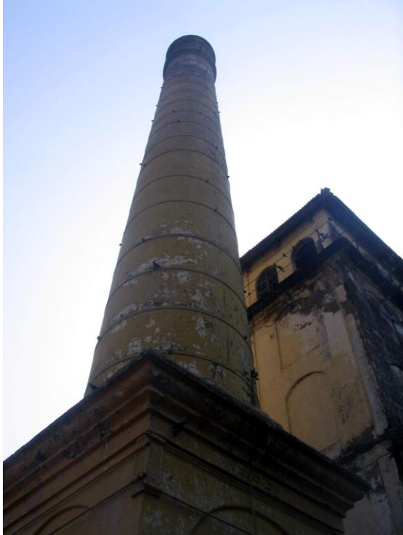
Goldmohur Mills - Chimney
