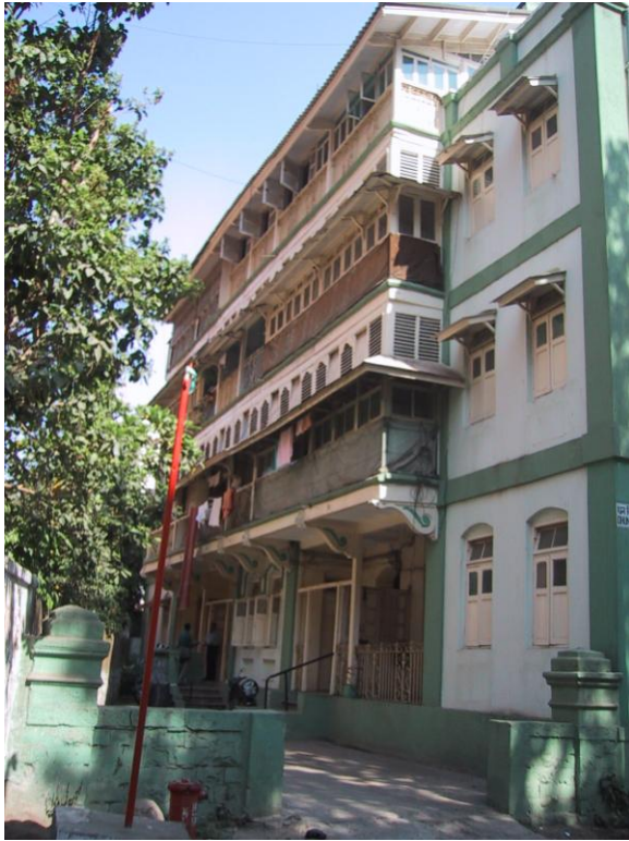
Elevation view of the building from Sant Gadge Maharaj Road
