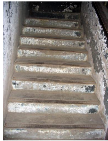
View of staircase
