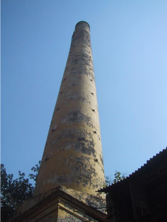
View of the Chimney
