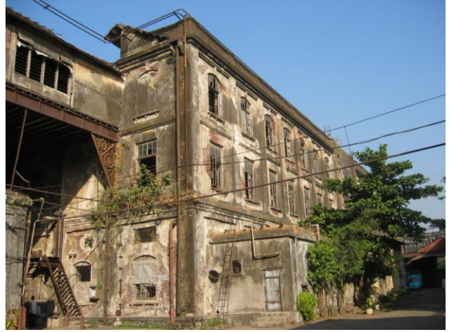
View of front facade
