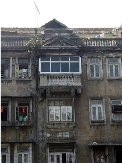
View of the Pediment on top floor
