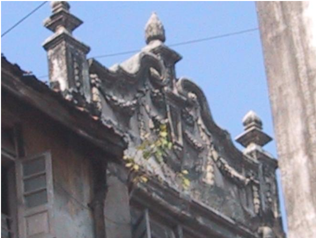
Detail on the top of the building
