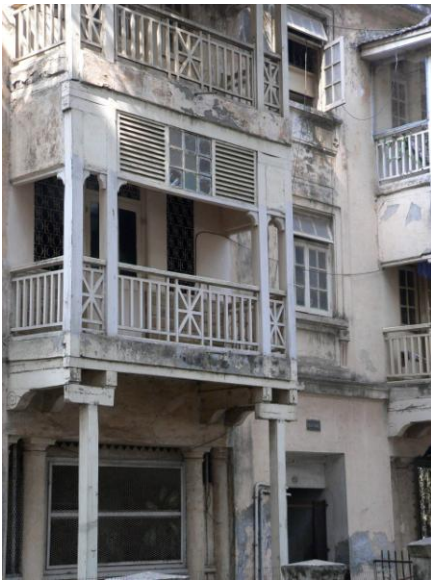
View of balcony detailing
