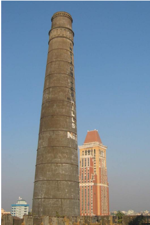
Chimney with newly built 'The ITC Grand Central Hotel' in background
