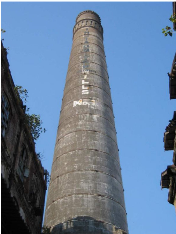
View of Chimney from below
