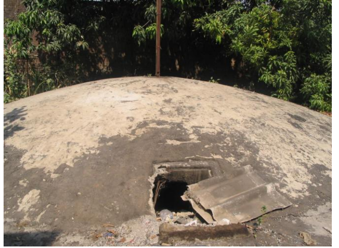
View of Oil Tank
