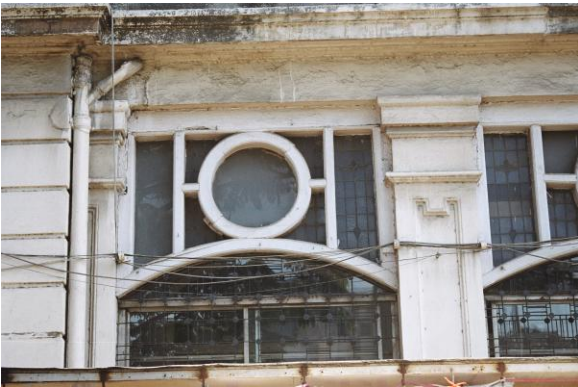
Stain glass provided for ventilators
