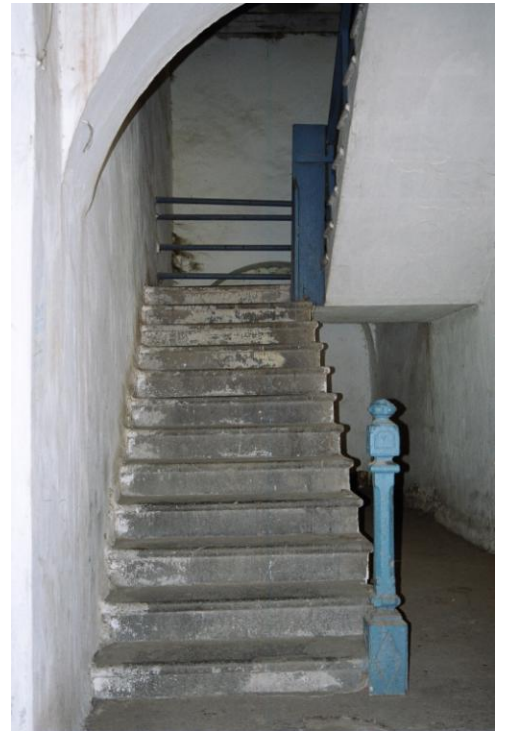
View of main staircase
