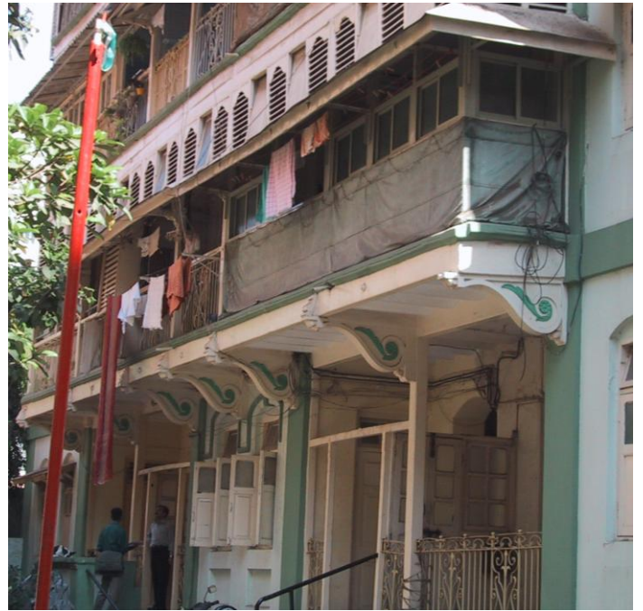
View of balcony detail
