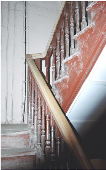
View of staircase
