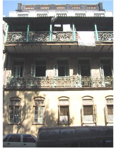
Highly decorated balcony railings
