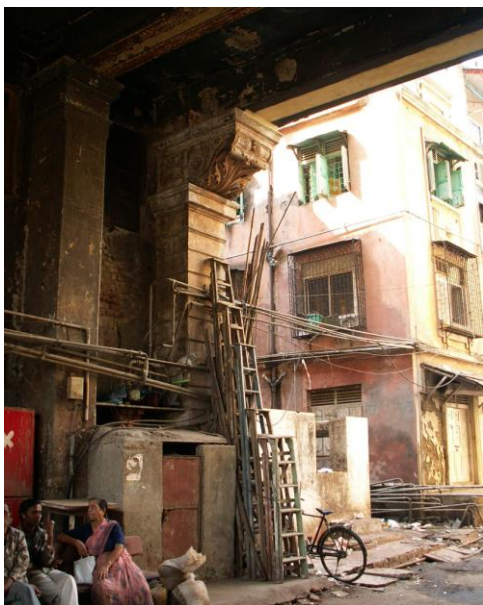
Details at the entrance gate
