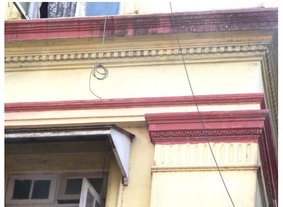
Decorative capital on the pilasters
