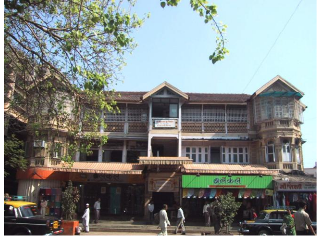
View of the building from Dadasaheb Phalke Road
