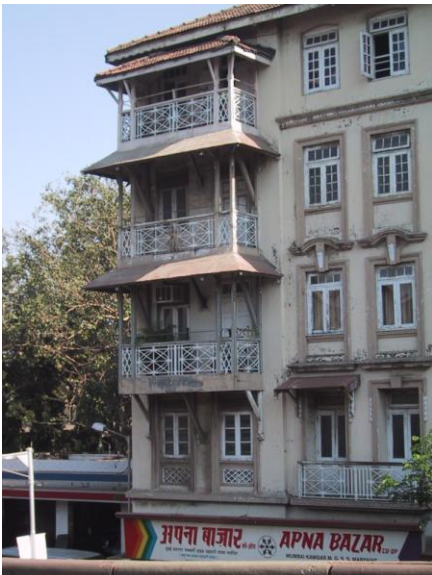
View of the balconies on front facade
