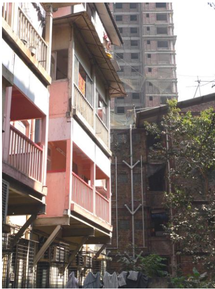
Internal balcony detail
