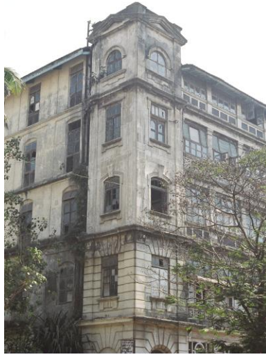
Stucco work on ground and first floor
