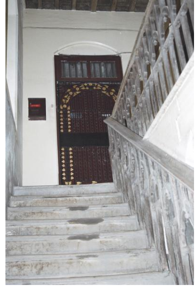
View of staircase
