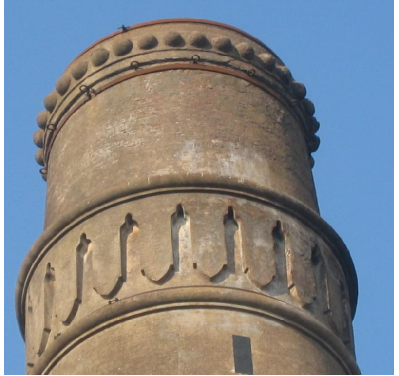
Detail of the chimney top
