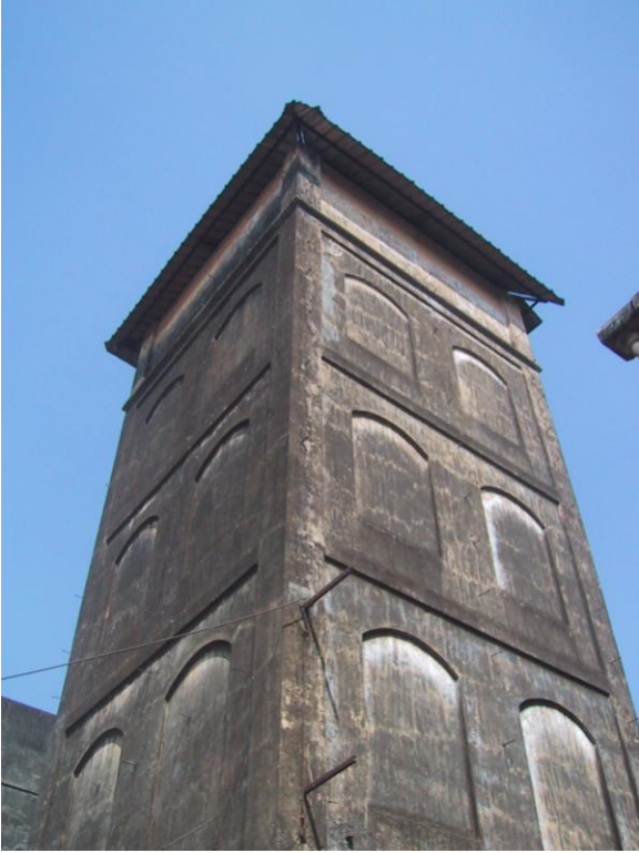
External view of Dust Chimney
