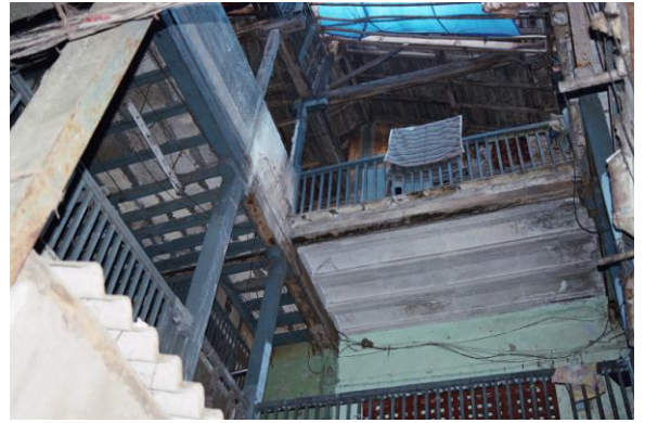
Main Staircase Shaft, with a cut out above
