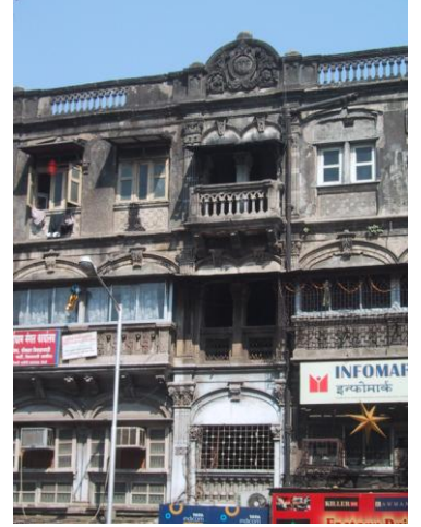
View of front facade
