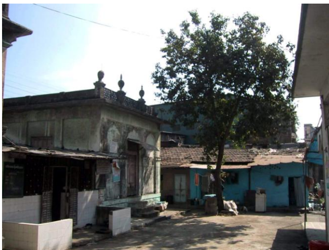
Internal view of complex from the entrance
