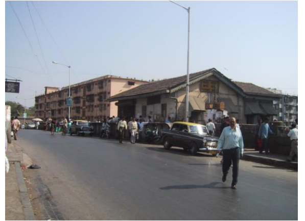
View of the bridge.
