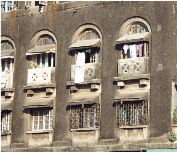
View of windows with semi-circular arches above
