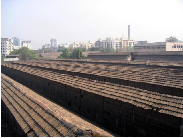
View of North Light Trusses
