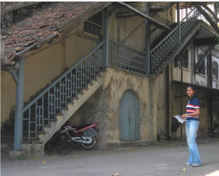
View of Wooden Staircase
