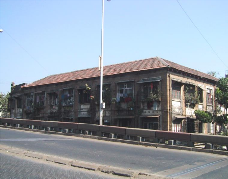
View from bridge at Parel junction on Dr. Babasaheb Ambedkar Marg
