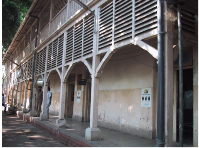
Wooden louvered ventilators
