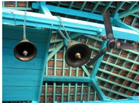
Roof detail with tiles laid directly over purlins on the truss
