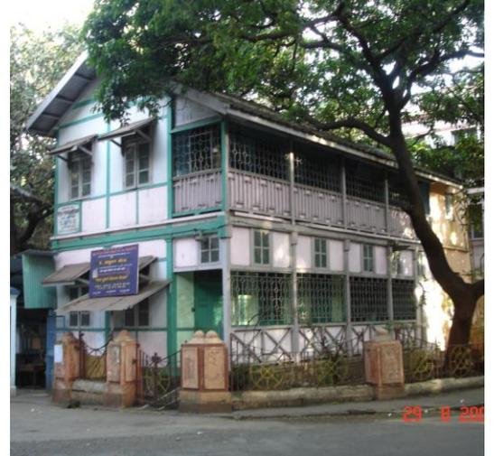
Modest scale building with timber structural members and brick filling with a road facing wooden balcony and sloping roof
