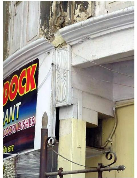
Detail of the load bearing wooden structural members near the staircase
