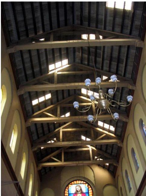
Original timber boardings removed and acrylic skylight along with asbestos sheet roof is an add-on
