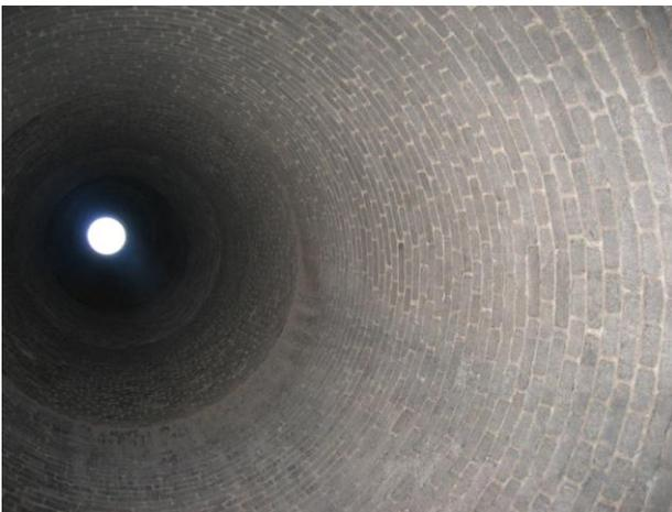
Interior of the chimney with construction of brick masonry in cylindrical profile
