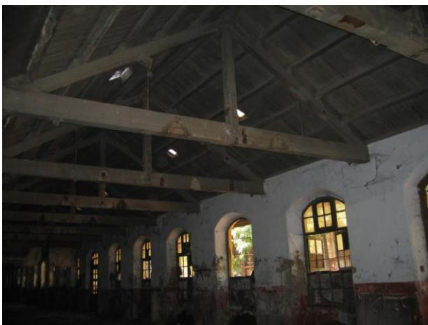
Segmental arched windows at equal intervals and detail of wooden roof trusses
