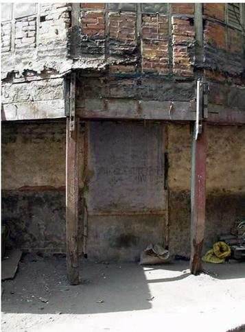
Extremely dilapidated structure supported on props
