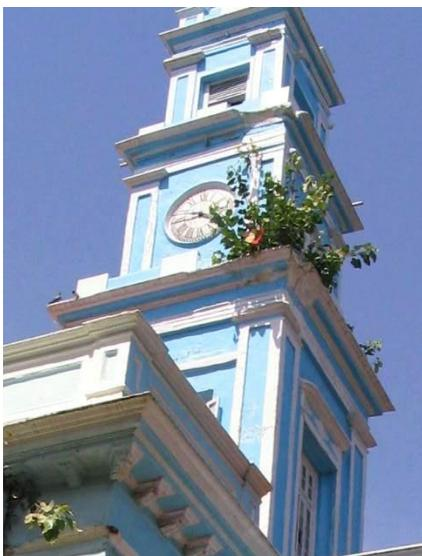
Horizontal bands on clock tower with beginning of tree growth on the tower
