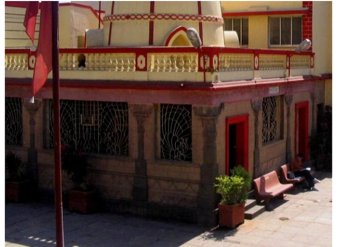
Façade with original carved stone pillars with newly constructed brick walls plastered & painted like Malad stone
