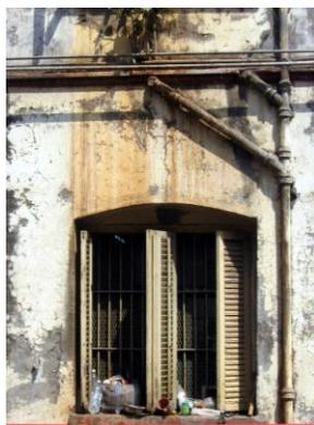
Leakage from the downtake pipes damage the plaster
