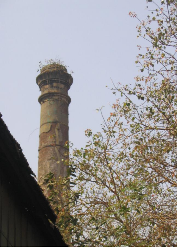
View of Brick Masonry Chimney with horizontal bands
