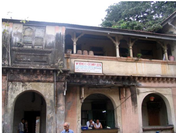
Semicircular arcade on the ground floor
