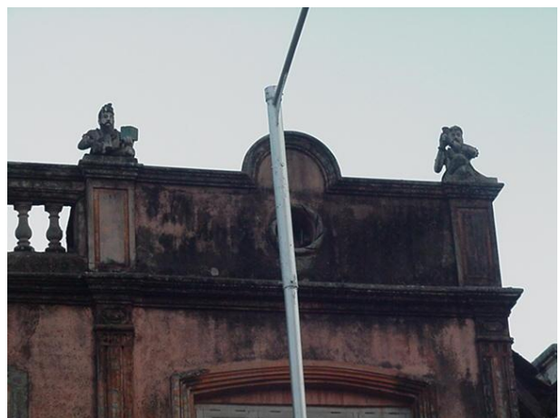
Decorative idols of God above the terrace parapet level
