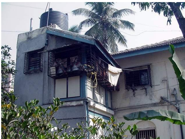
Overhead water tank
