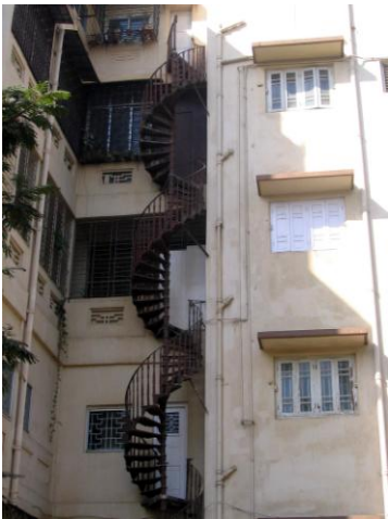
Cast iron spiral staircase
