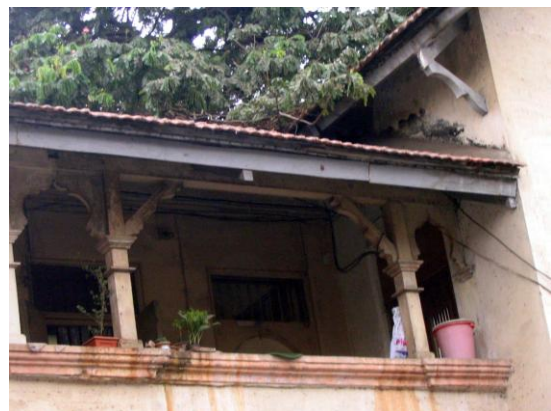
Cill of the parapet has a moulding
