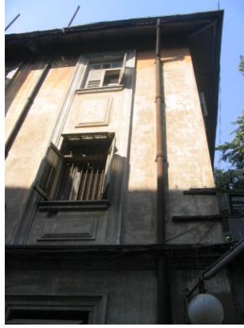
Plain façade of the structure facing S.K Bole road
