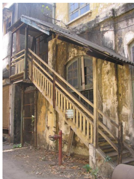
External staircase to folding department
