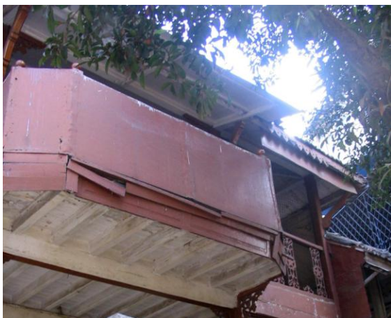
The balcony requires maintenance
