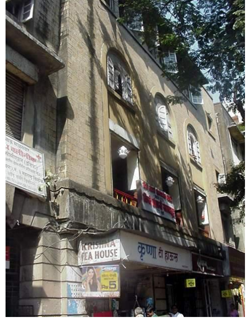
Malad stone cladded façade
