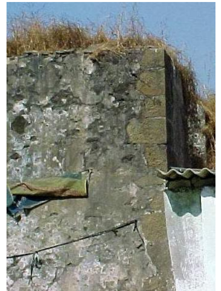
Malad stone dressed masonry for the corner junction
