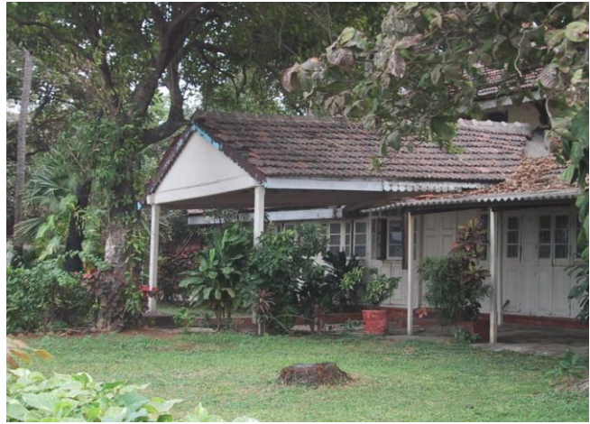
Large porch with Mangalore tiled sloping roof and landscape give ambience of a bungalow
