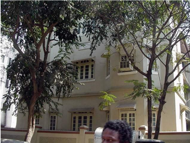
View of the side façade
