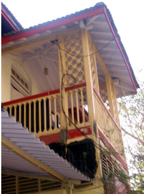
Projecting balcony with simple balusters
