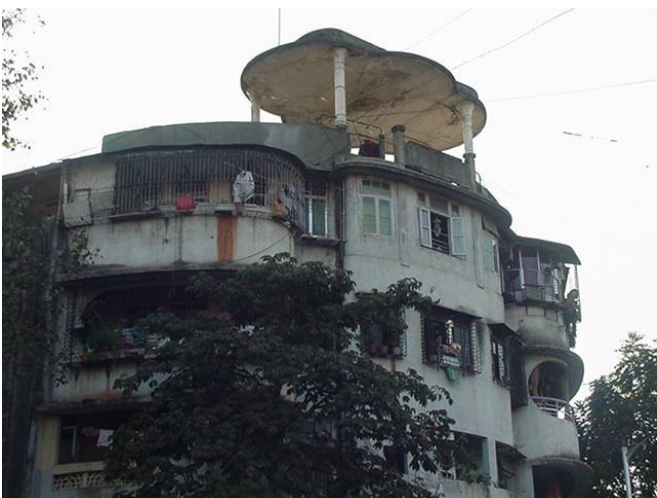
Corner terrace has a flat roof supported by reinforced columns
