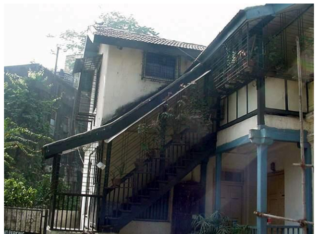
External staircase covered with a roof
