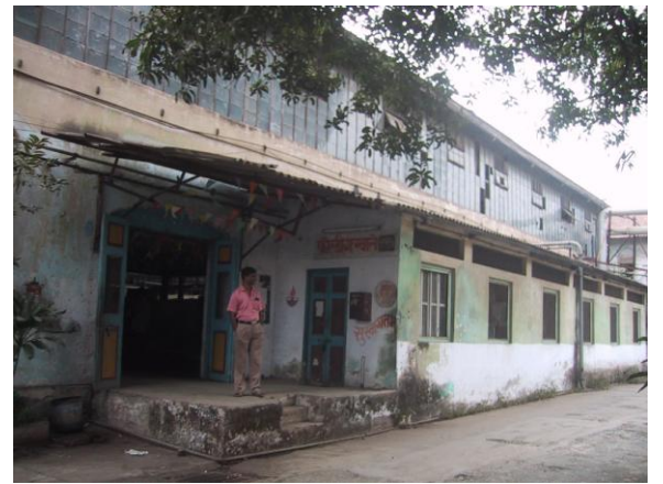
View of elongated façade of the Folding and Finishing Department
