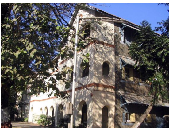
Façade facing the playground
