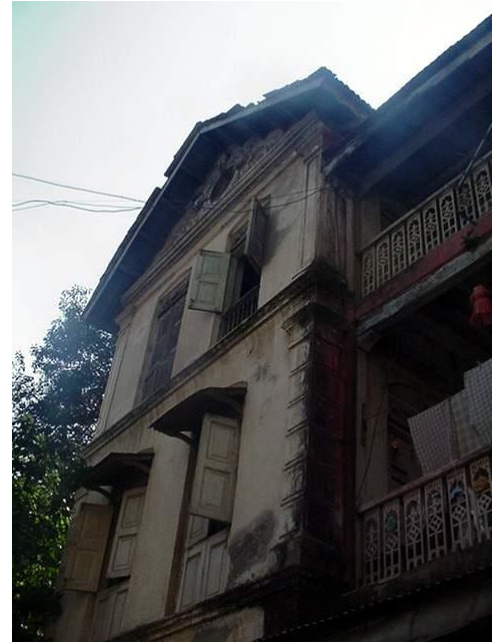
View of the elevated bay
