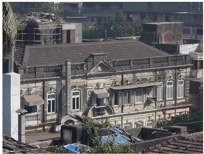
View of the whole façade
