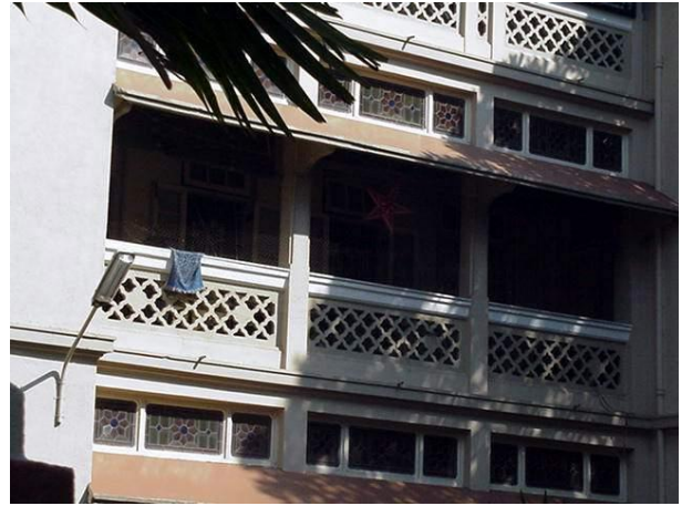
Criss cross concrete jali at the parapet
