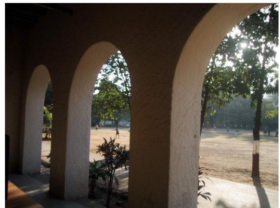
Semicircular arcade on the ground floor
