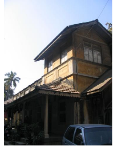
G + 1 structure with lean to roof on the ground floor
