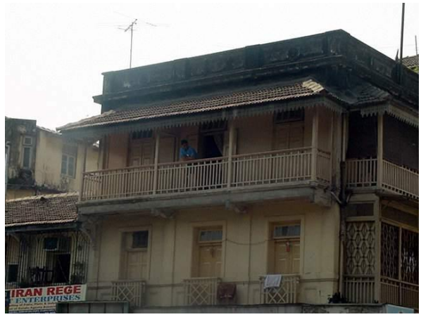
Projecting balcony on the 1 st floor
