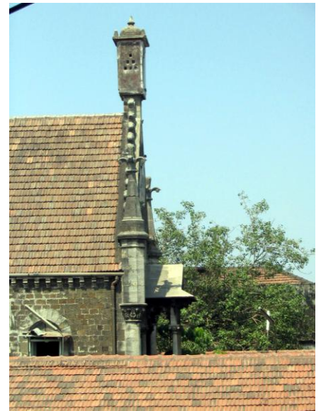
Decorative roof gable
