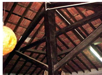
Wooden king post truss
