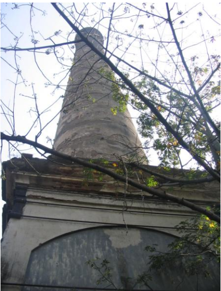
Brick masonry Chimney with base having cornice band
