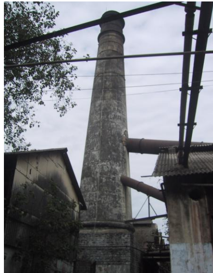
Brick Masonry Chimney with Boiler Room
