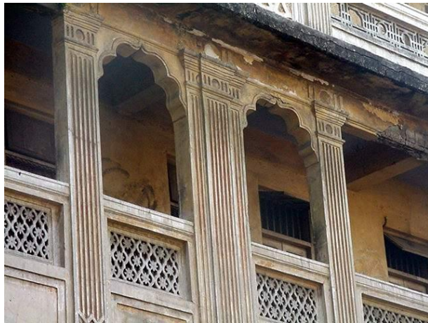
Decorative arches in between grooved pilasters
