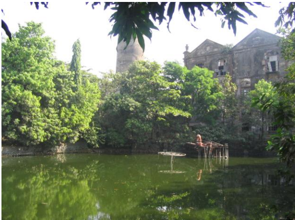
View of Blow Room and Mixing Department and lake in the foreground
