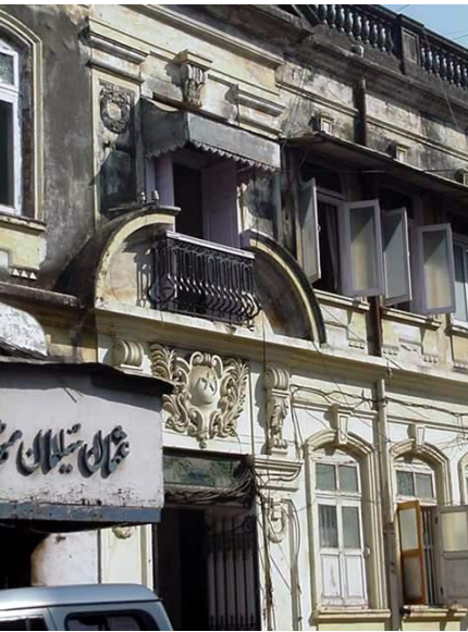
Windows have decorative architraves with key stones
