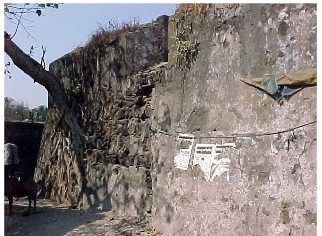
Fort wall in Black Basalt random rubble masonry
