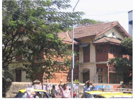
View obstructed by vegetation
