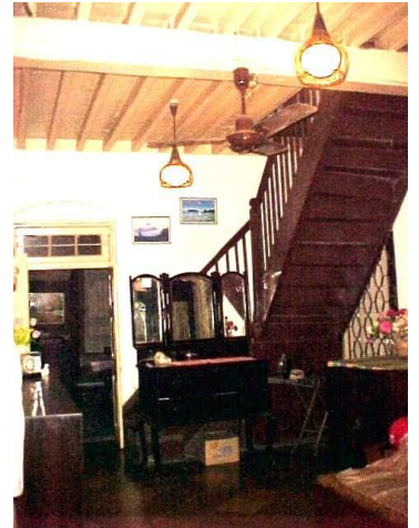
Internal straight flight staircase
