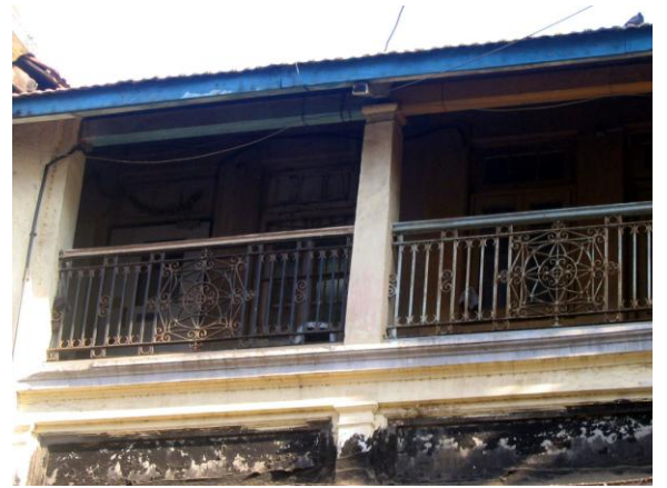
Balconies with simple balusters
