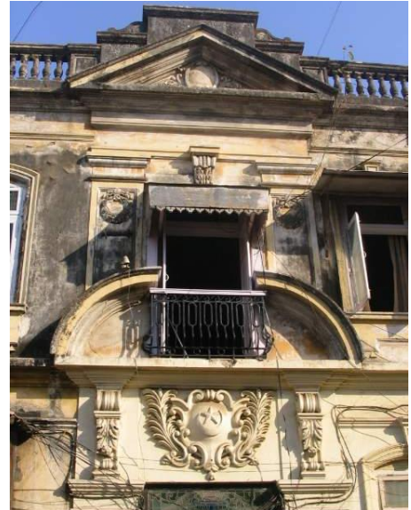
Neo-classical details on the façade
