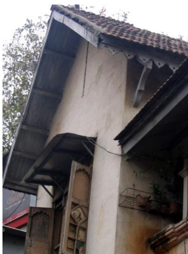
Plain eaves fascia
