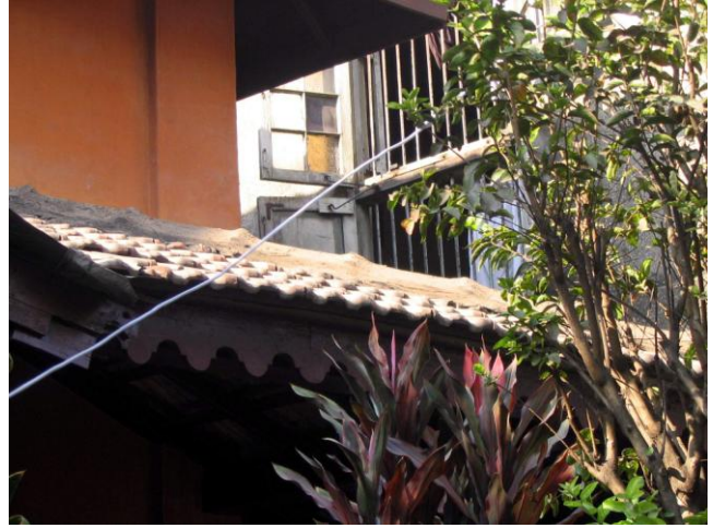
Detail of eaves
