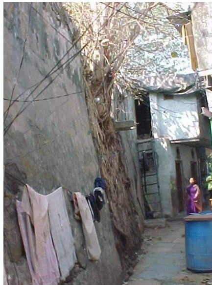
Slums and tree growth on the south-eastern walls of the fort
