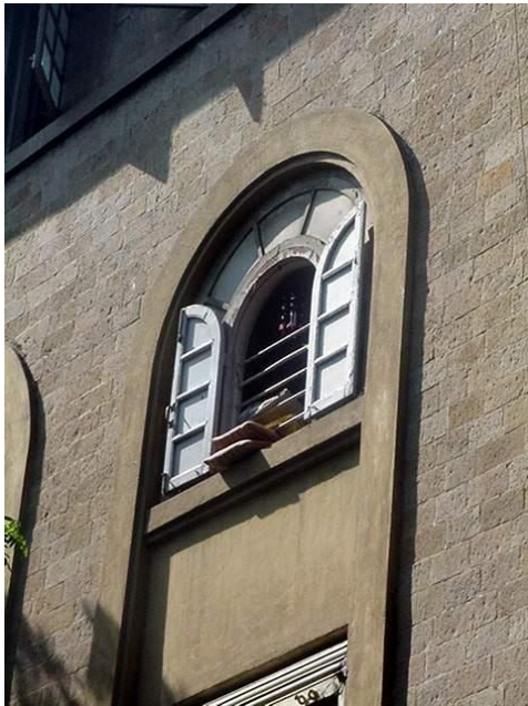
Semicircular opening with simple architrave
