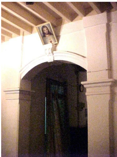
Wooden joist flooring
