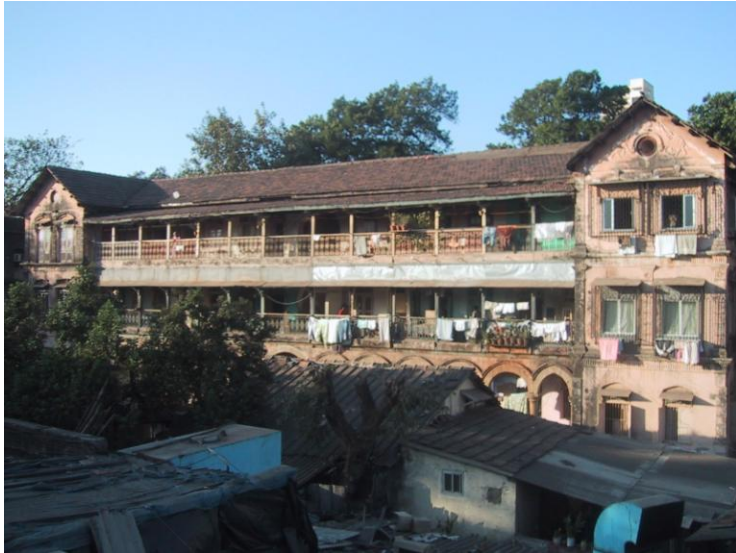
View from Matunga flyover
