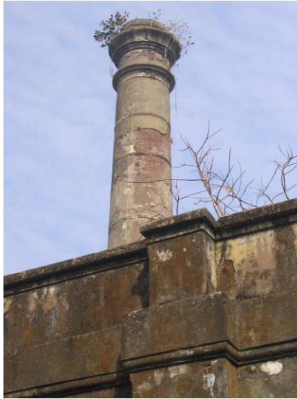
View of Chimney from the mill premises
