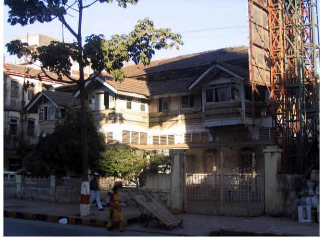
A huge commercial banner stands at the left side of the building
