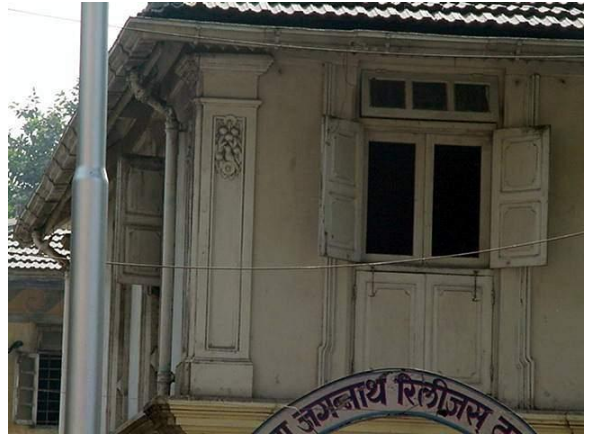
Decorative pilasters on the façade
