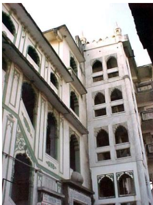
View of the internal façade
