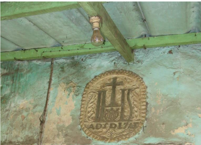
Date encrypted on the wall
