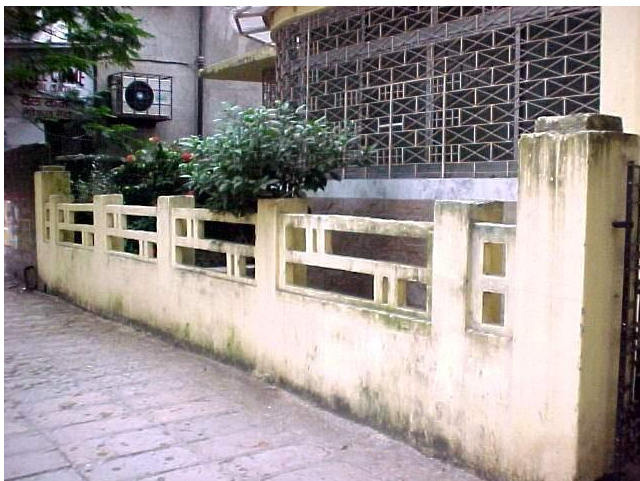
View of the compound wall
