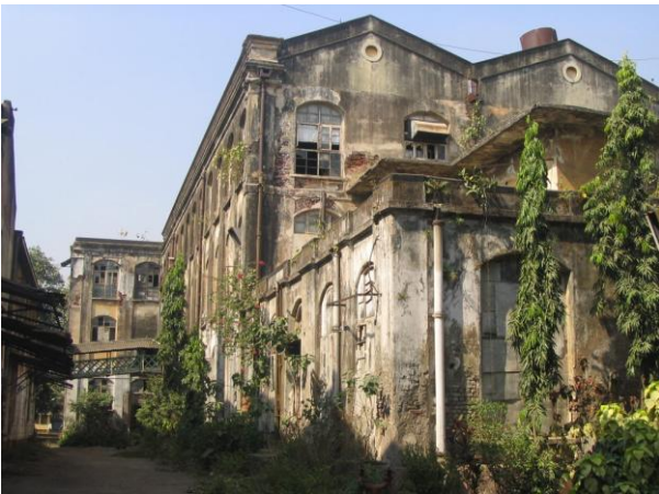
Vernacular style elongated façade of Card Department
