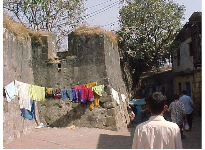
Side walls of the fort, now in ruins
