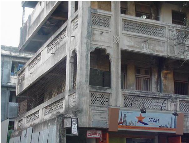
Decorative concrete jali at parapet level
