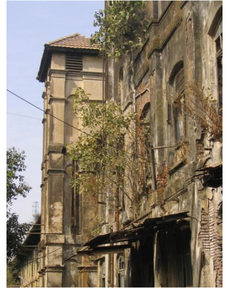
Vernacular style façade with horizontal bands & segmental windows
