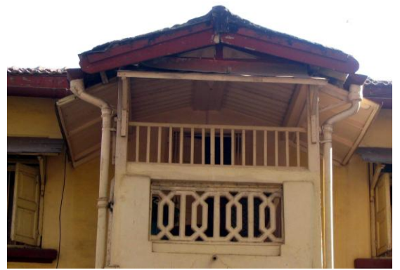
Downspout pipes from the gutter
