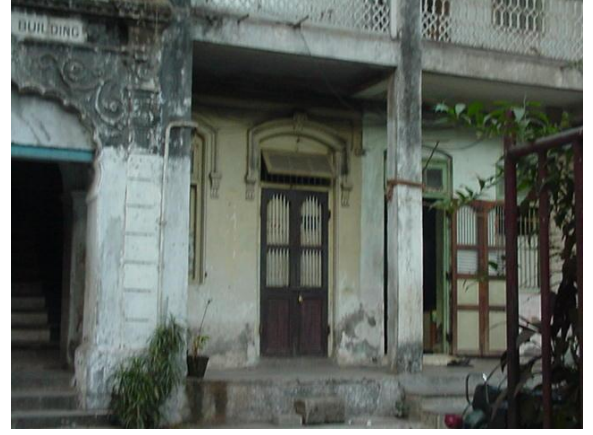
Decorative architraves around the doors of the verandah
