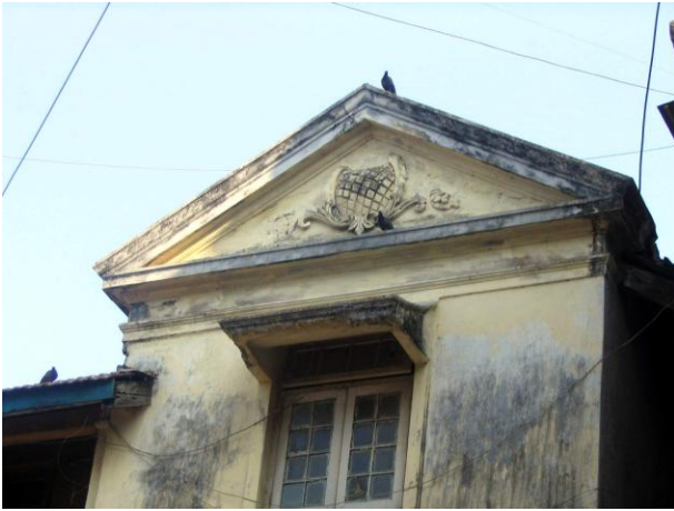
Triangular parapet wall with decorative motifs
