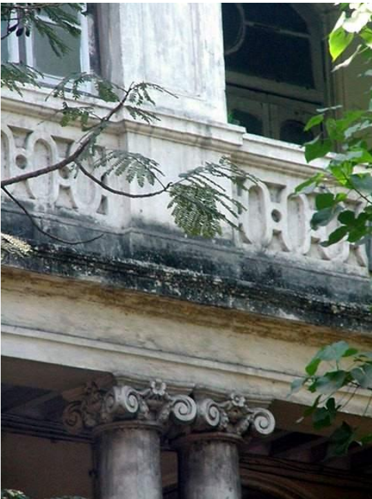
Decorative concrete jali at the parapet level
