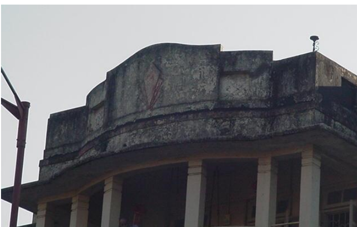
Decorative parapet wall
