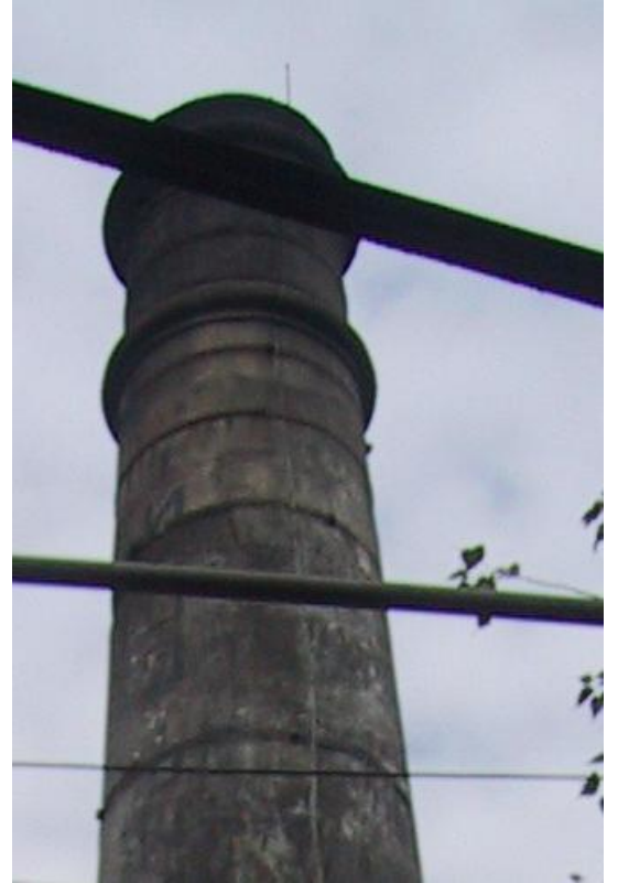
Brick masonry chimney with horizontal bands at the top portion
