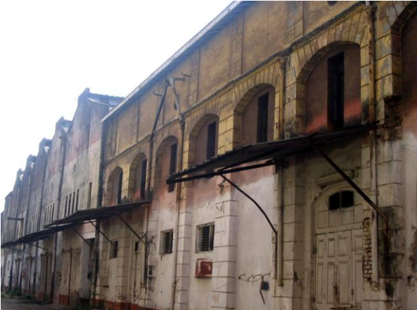
View of Weaving Shed
