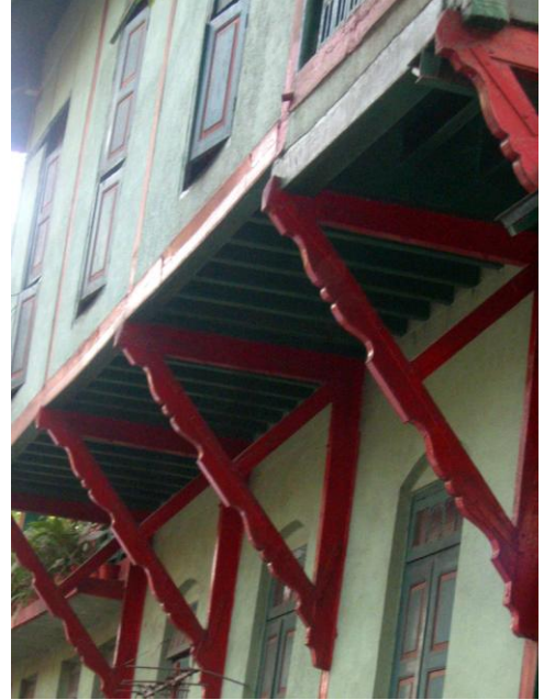
Oil painted carved wooden brackets
