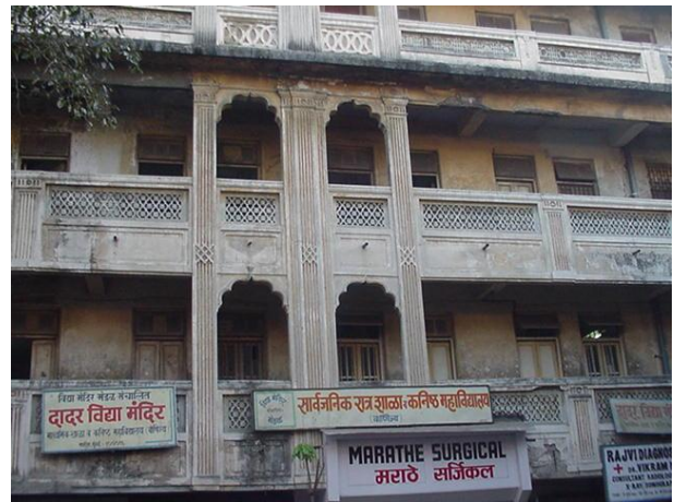
Ground floor has commercial sinages
