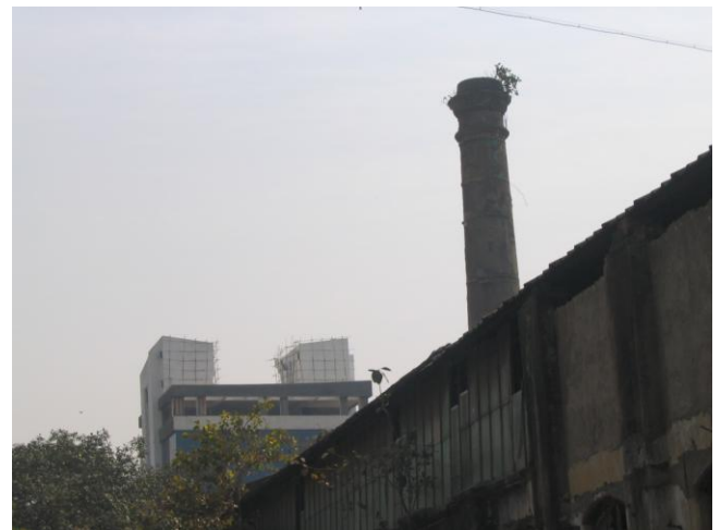
View of Auto loom shed and Chimney
