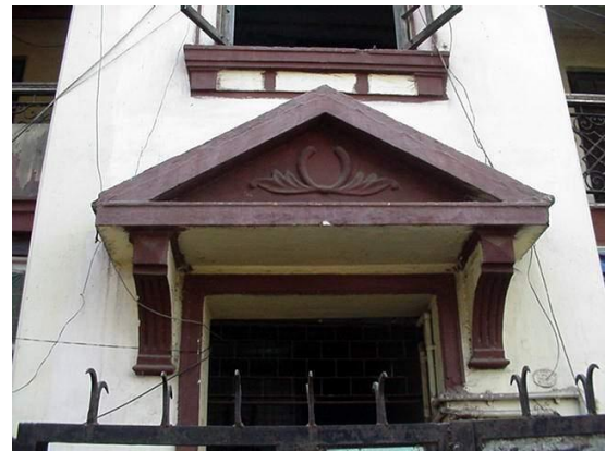
Triangular element above the entrance
