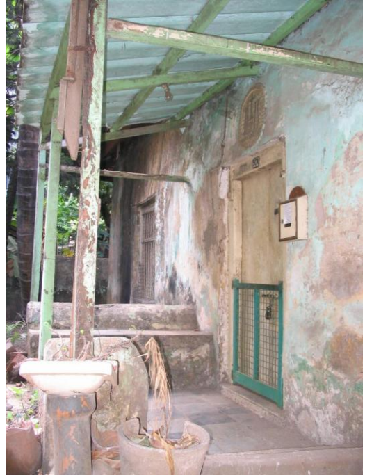
Verandah on the external side of the bungalow
