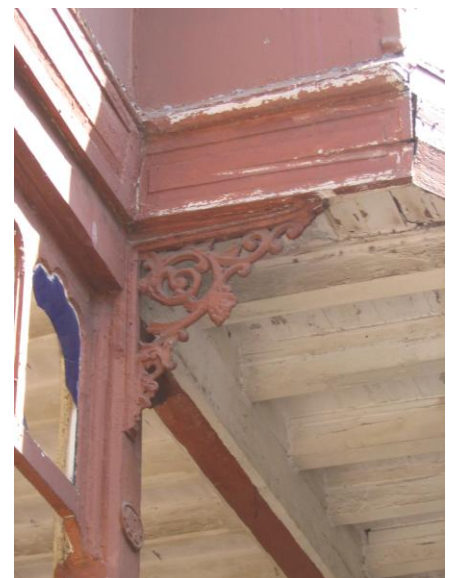
Decorative cast iron brackets
