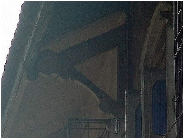
Decorative wooden brackets supporting the roof
