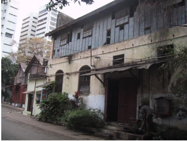
View of Plain façade with North light truss
