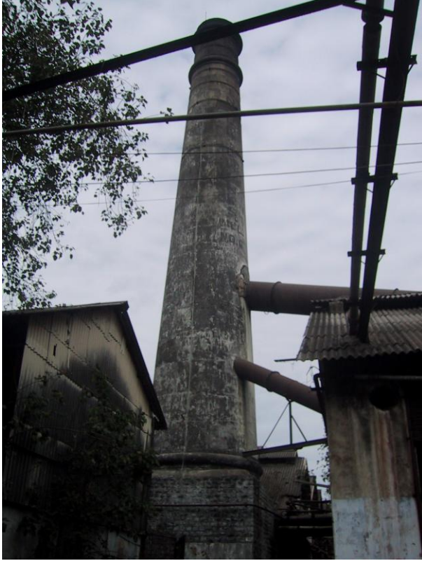
View of brick masonry chimney with boiler room
