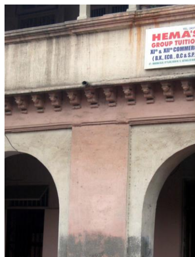
Cornice band supported by decorative corbels
