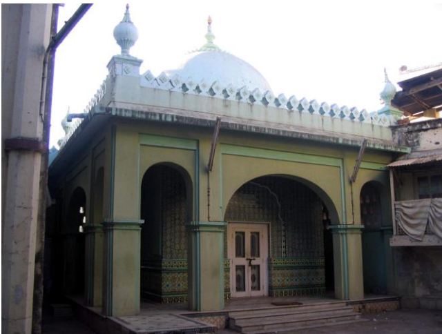
Internal shrine of the premises
