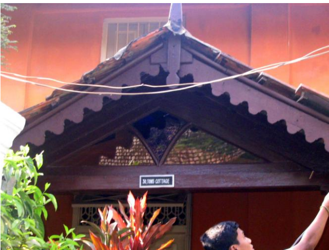
Roof detail of the entrance porch
