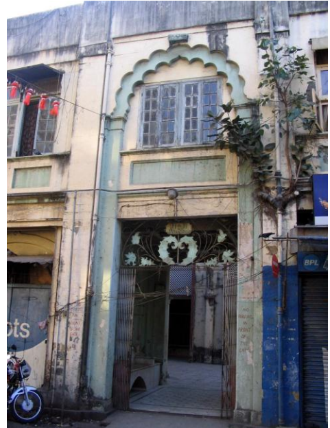
Mughal arch in stucco work for the entrance
