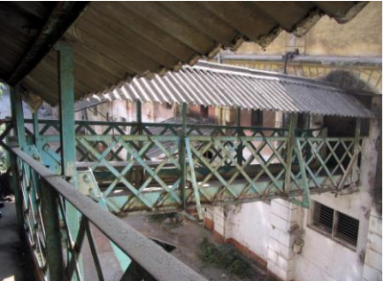
M.S. bridge connecting two structures
