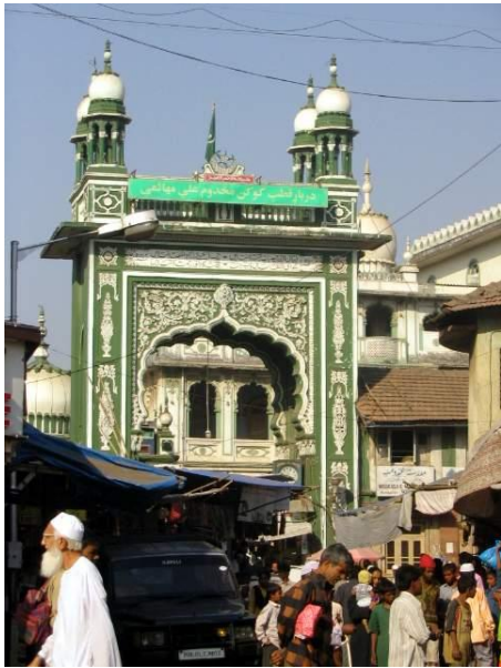
View of the entrance gate
