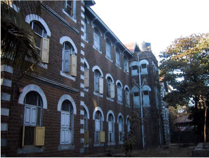
Façade facing Matunga railway station
