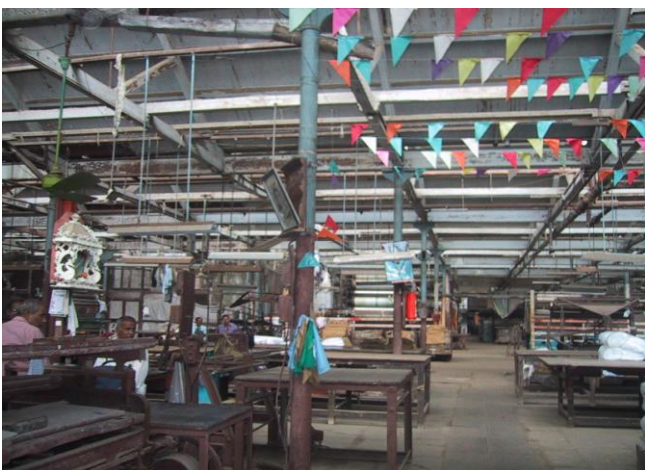
Internal view of the Weaving Shed
