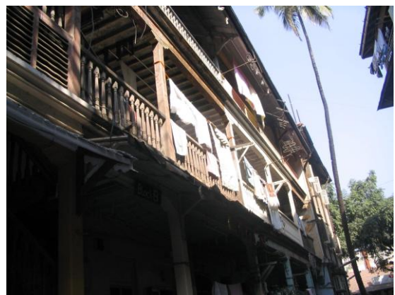
Long stretch of balconies used as common corridors
