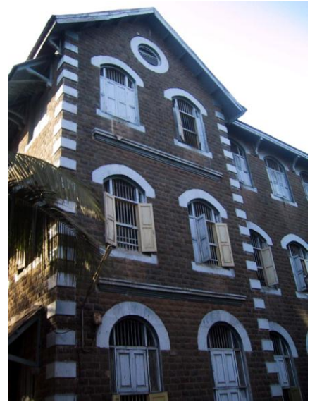
Black Basalt with highlighted arches and long and short work at the corner edges of the building
