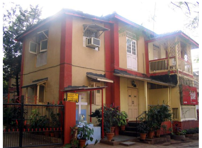
View of the front façade
