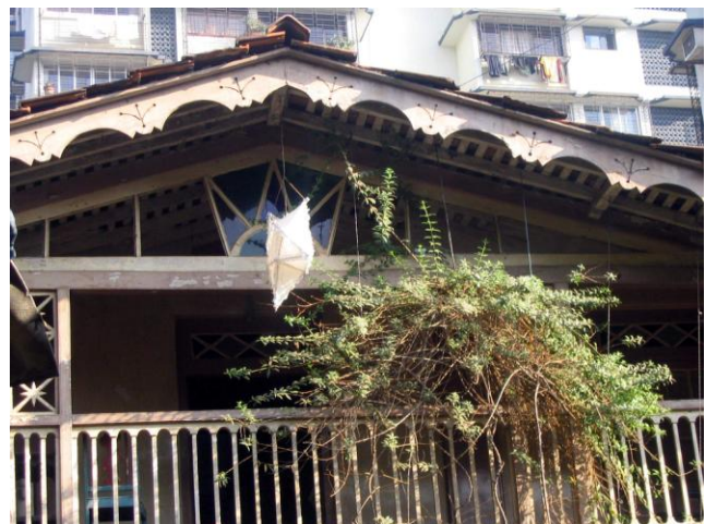
Decorative wooden eaves fascia
