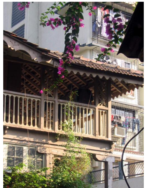
Balcony having simple wooden balusters
