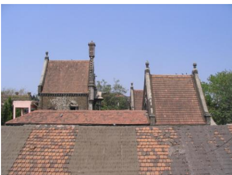
Roof profile of the hostel
