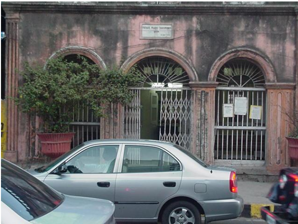
Collapsible grills seen on the ground floor
