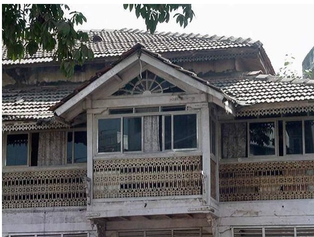
Cantilevered balcony with a sloping roof
