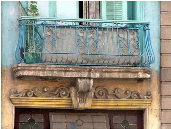
Decorative floral motifs in stucco work above the architrave
