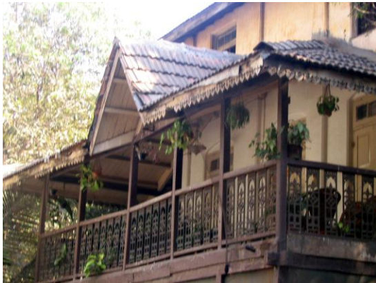
Pitched roof for the projecting balcony
