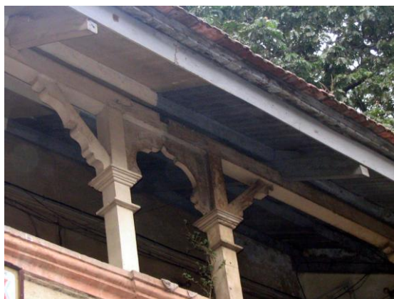
Decorative wooden posts and carved brackets
