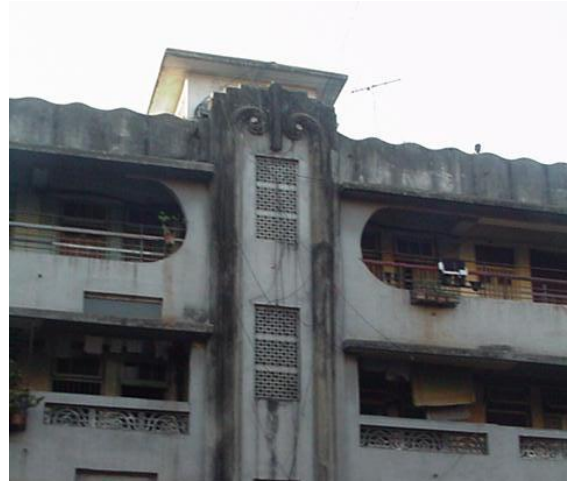
Decorative terrace parapet wall
