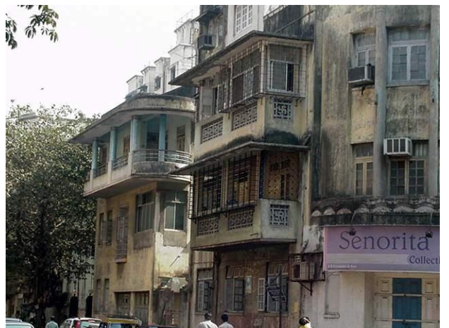
Shopline on the ground floor
