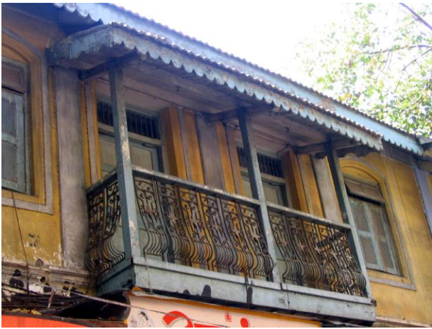
Balcony supported by wooden posts
