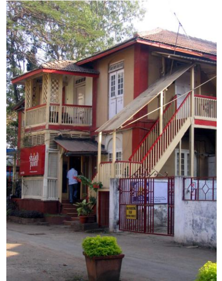
External straight flight staircase
