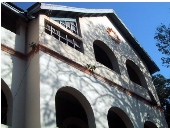
Plain façade with semicircular cut outs
