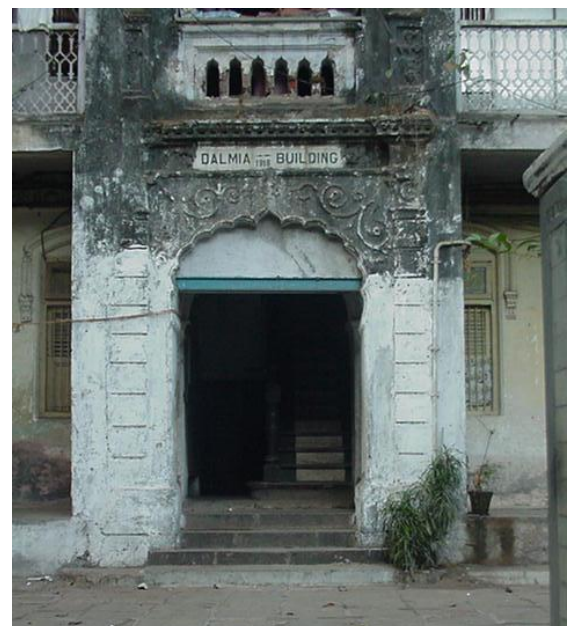
Decorative motifs above the entrance arch
