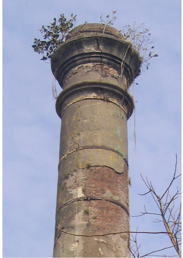
Plaster chipped off and tree growth on façade of chimney
