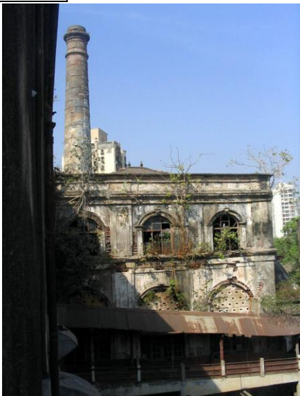
View of Production Department and Chimney
