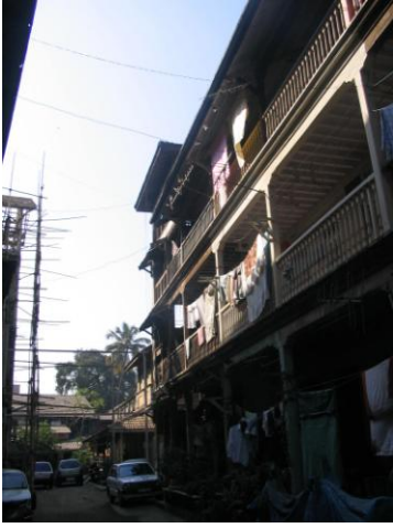
View of one of the buildings of the premises
