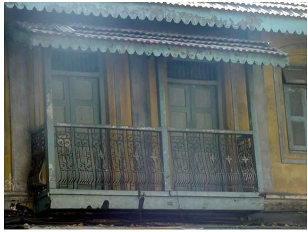
Decorative cast iron railing
