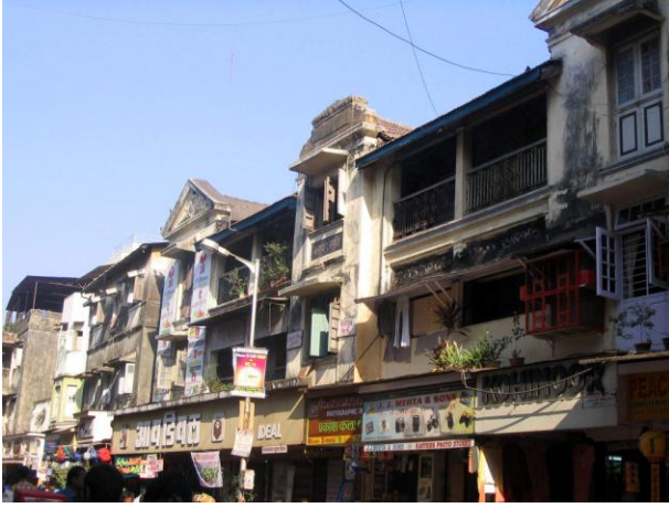
View of the façade from Chabildas Road
