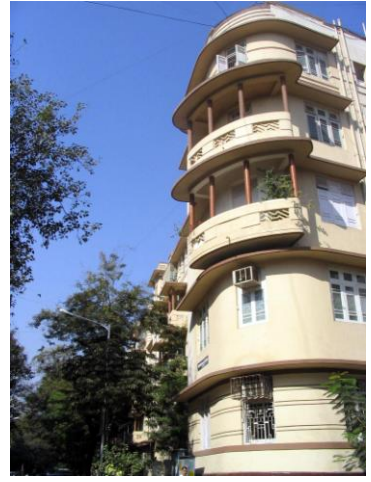
View of the corner building
