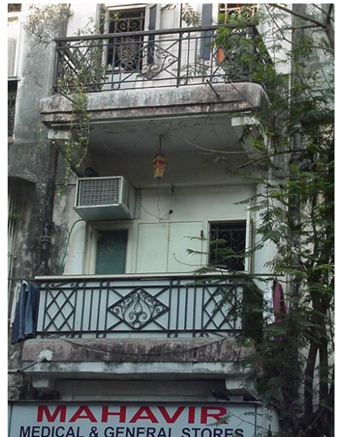
Decorative cast iron railing
