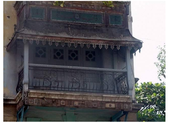
Sloping roof chajja for the projecting balconies
