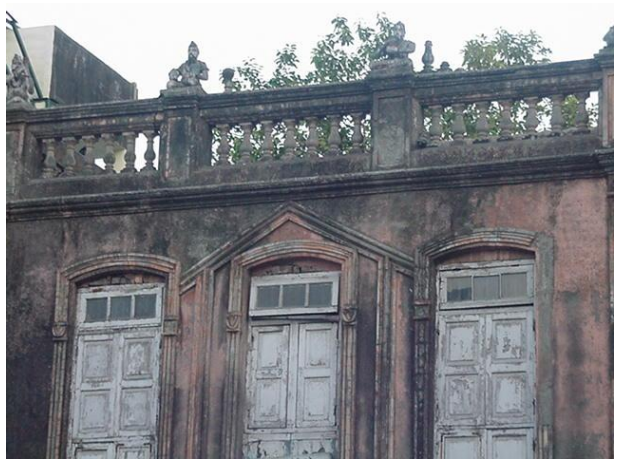
Decorative concrete jali at the terrace parapet level
