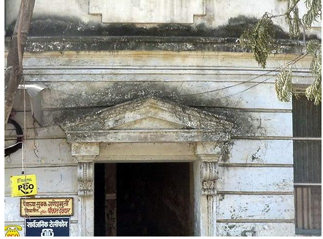
Decorative consoles below the pediment
