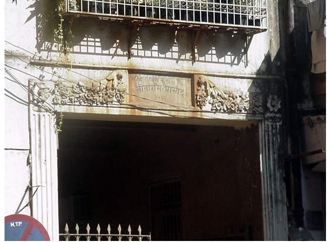
Floral motifs with fluted pilasters for the entrance porch
