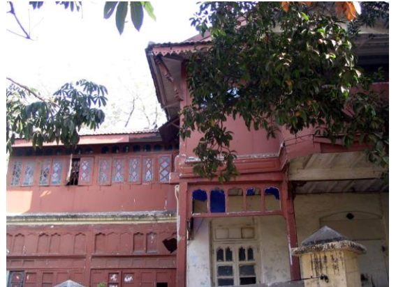
The maroon colour of the façade highlights the structure
