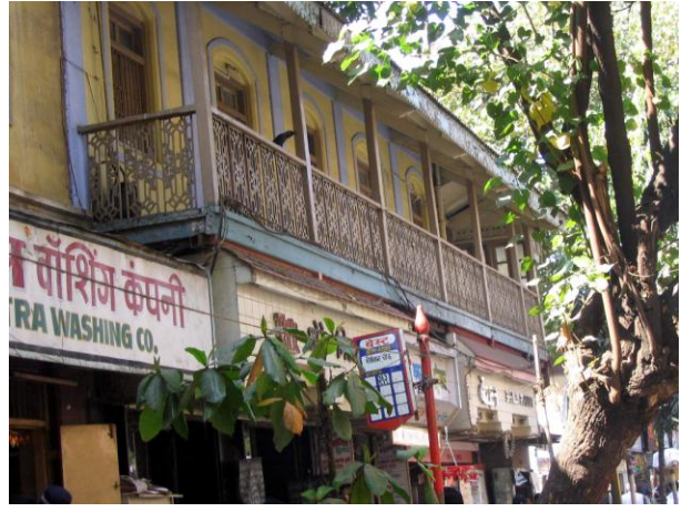
View of the projecting balcony
