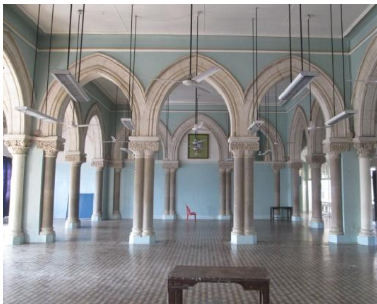
BJPC School after restoration
